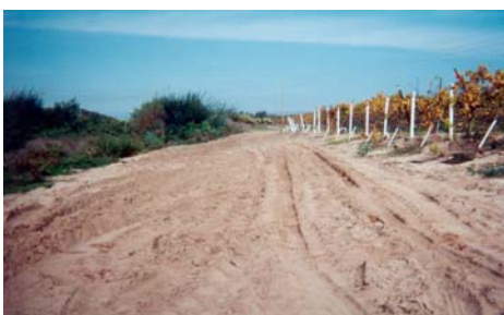
(Demo Area Prior to BMP)
